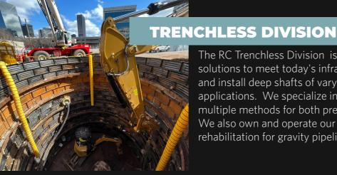
The RC Trenchless Division is capable of performing a multitude of solutions to meet today's infrastructure challenges. Our team can dig and install deep shafts of varying diameter to support many trenchless applications. We specialize in tunnel and horizontal boring utilizing multiple methods for both pressure and gravity pipeline applications. We also own and operate our spiral wound PVC lining equipment for rehabilitation for gravity pipeline applications.
